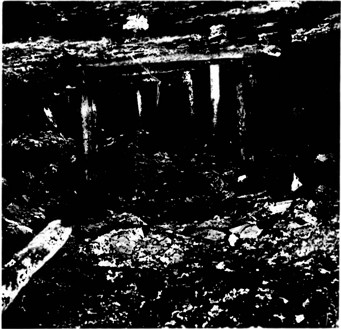
FIG. 10. Typical Temporary Coal Mine Opening After 10 Years of Disuse. In this instance it is located 240 feet beneath the sea floor, with a water cover of 60 feet (Dominion Coal).
